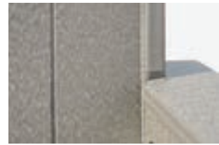
State of the art welded seams
